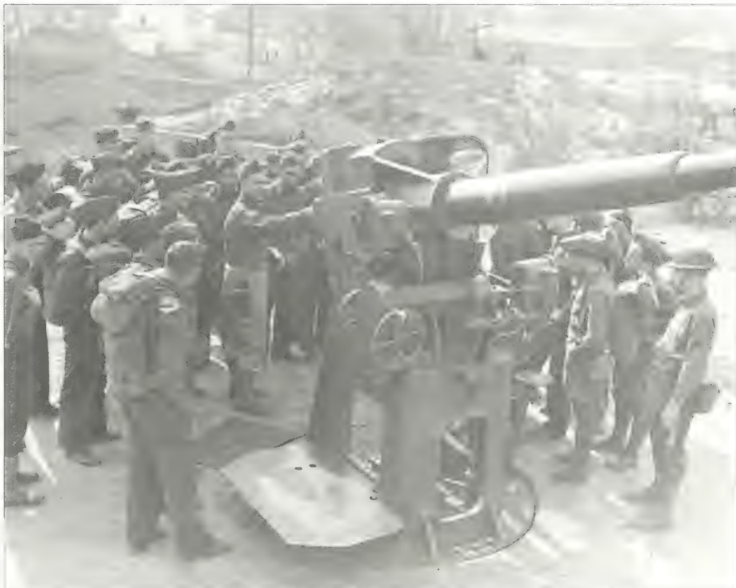
Figure 2.69. View looking southwest at anti-aircraft gun on top of the Mortar Battery, circa 1941. With the start of World War II, the anti-aircraft guns were supplemented by a machine gun platform. A .50-caliber machine gun is visible in the background and the base of the Sandy Hook Lighthouse can be seen in the upper left (GATE 7588).
